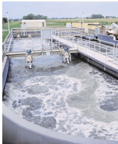
A ditch close-up shows bridge-mounted units.
