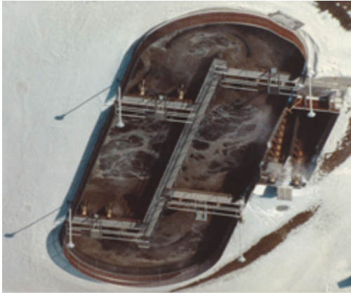
An aerial shot of the Madison oxidation ditch.
